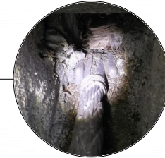
INTERIOR PHOTOGRAPH TYPICAL SUSPENDER CABLE & SEAT NOT TO SCALE
